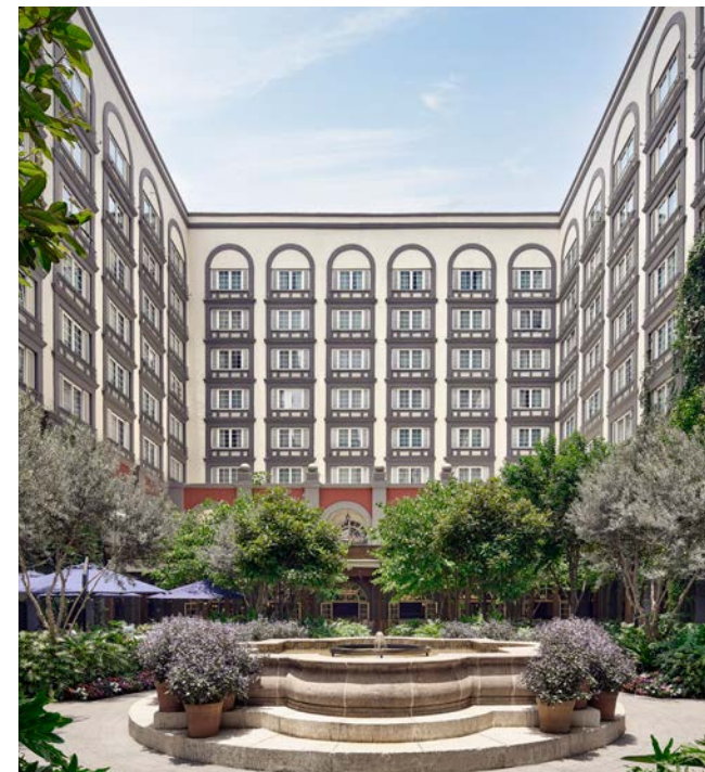
Four Seasons Hotel Mexico City courtyard
