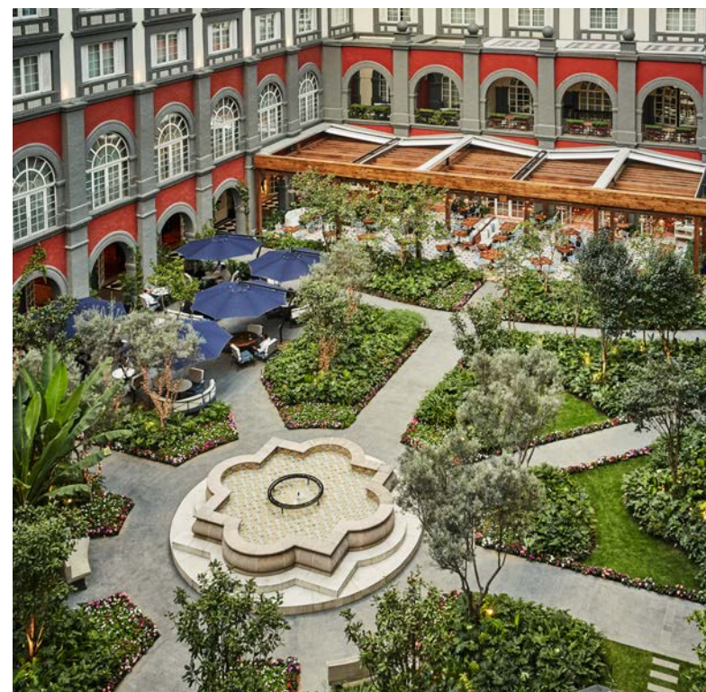
Four Seasons Hotel Mexico City courtyard
